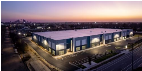
Northeast Business Center, Minneapolis, MN
